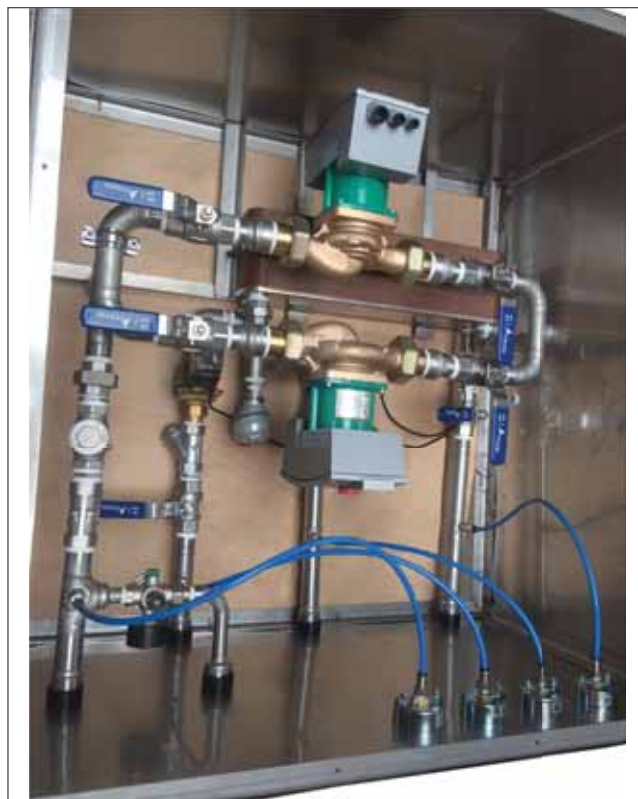
Circuit breaker between units with chiller.
